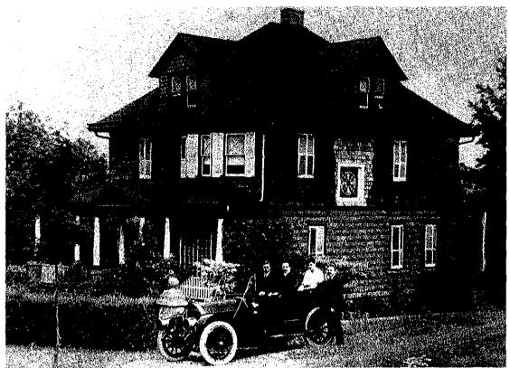
The lower story of this house at Madison Avenue and Eighth Street, still standing, was constructed of cement blocks manufactured in Cresskill. This type of construction was typical of the period. This picture was taken around 1920.
